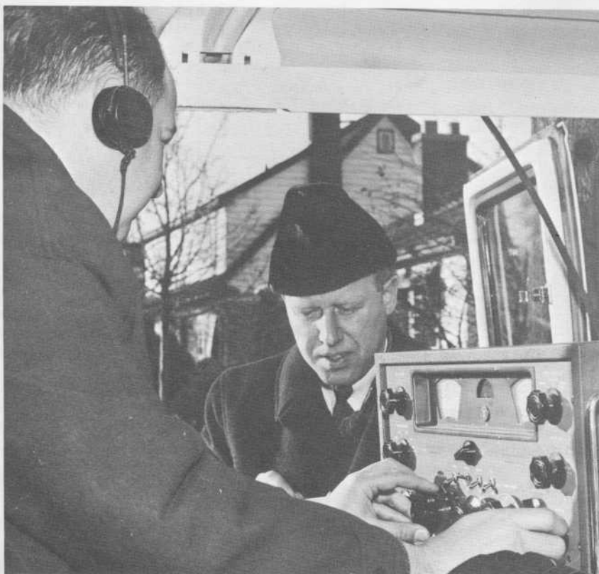
In 1930 Ralph Bunt, above, investigated radio interference with the aid of headphones, a portable receiver and loop antenna. Today John Demers (in fur hat) and Bob Coxe, Ottawa, are shown, left, tracing sources of interference by means of an all-wave communications receiver mounted in a specially-constructed radio van.
