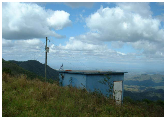
The abandoned cement hut on Vista el Mar.
